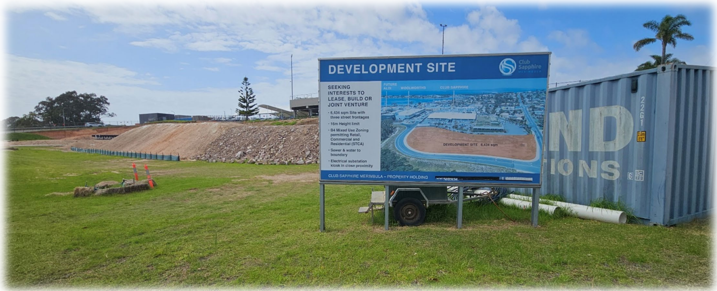
Development Site January 2025
